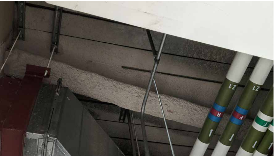
EXISTING CEMENTITIOUS FIRE PROTECTION
