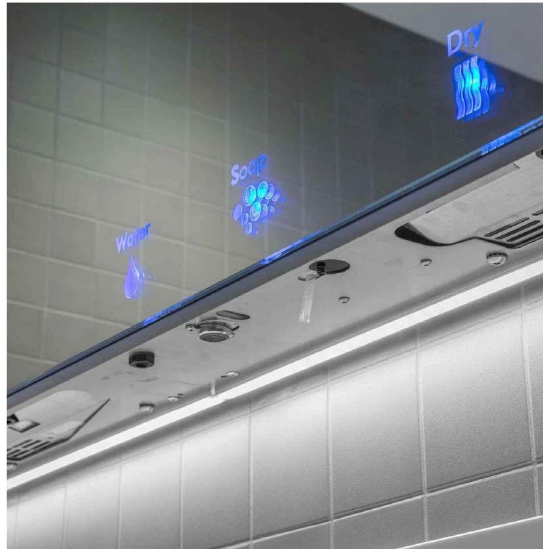
Continuous, solid-surface counter with individual sinks and bin shoots. Overhead mirror with integrated PIR activated soap and paper towel dispensers. PIR wall-mounted taps.
