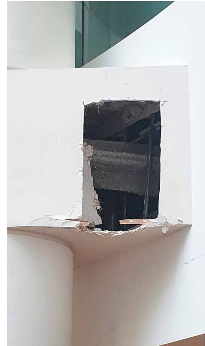
EXPOSED STRUCTURAL CONNECTION WITH FIRE PROTECTION
