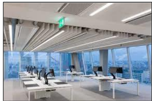
Chilled Beam with Acoustic Absorption
