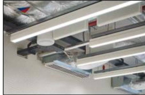
Vertical Acoustic Baffle
