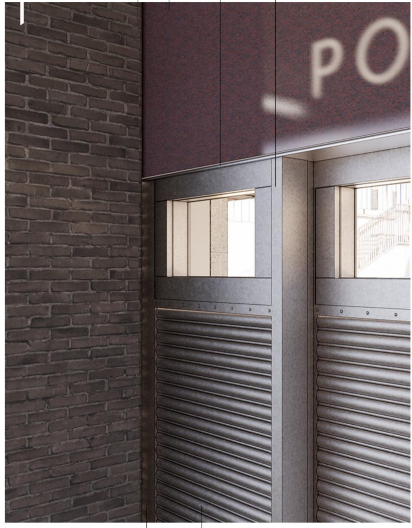
LIN-61: Galvanized steel straps, as part of overcladding to DRS-07.
